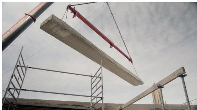
Figure 3.3 : Reuse of floor elements Prinsenof A (Retrieved from: Perree, 2022)
