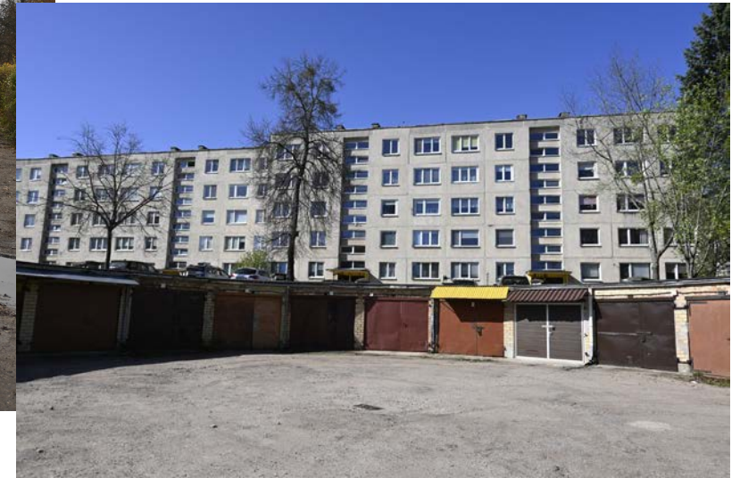
Fig. 62-63: Showing point M and N. Both images illustrate garages, with one featuring a round design, while the other presents a linear volume configuration.
