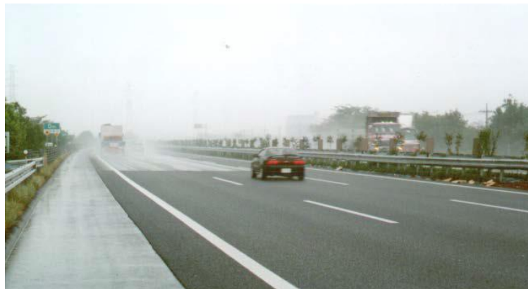
Figure 14, porous pavement and conventional pavement (Kubo, nb).
