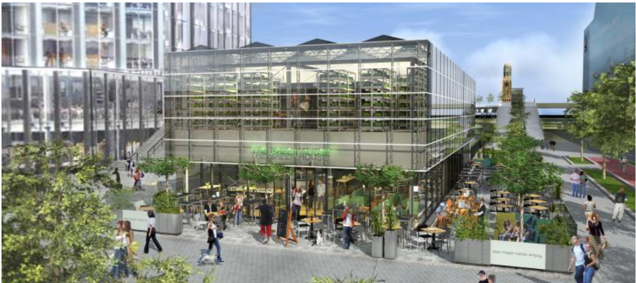
Figure 7.1: Circular Pavilion ‘The Green House’ Utrecht (The Green House, 2018)
