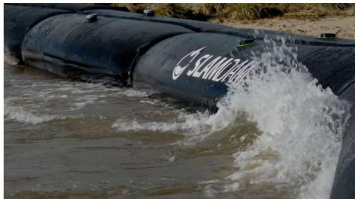
Figure 21: Slamdam: temporary flood defence that is filled with water (Slamdam (2019)).
