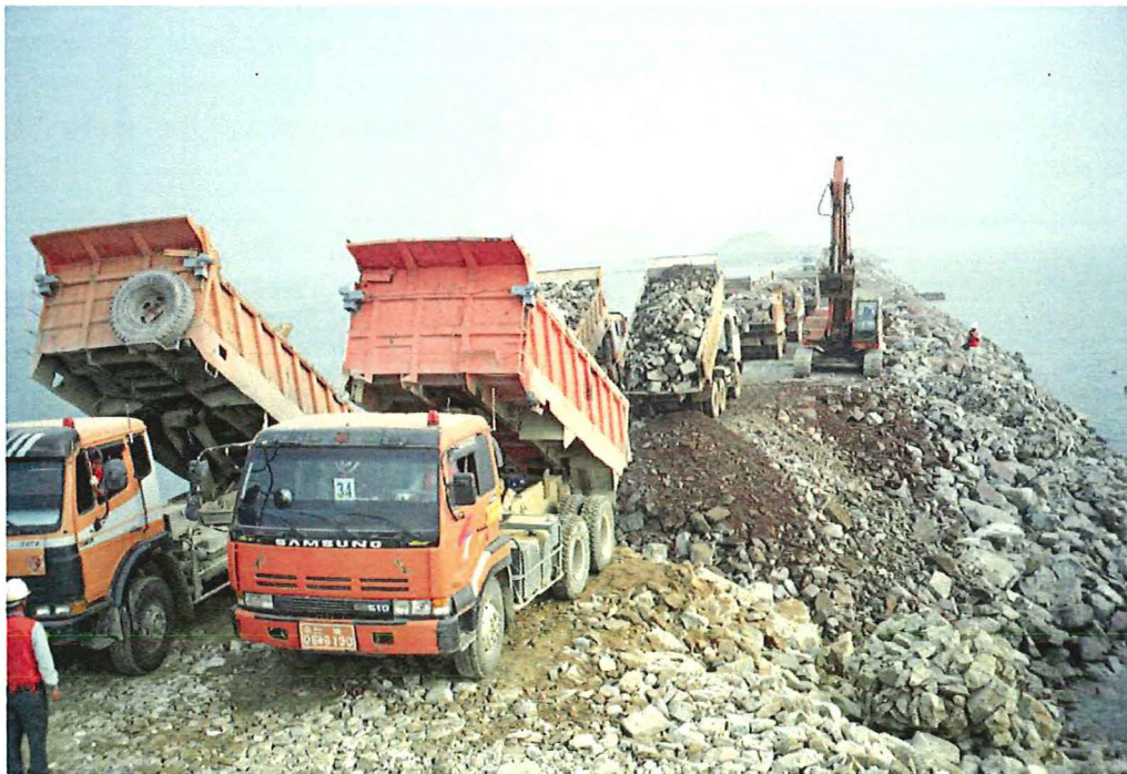
Figure 2.4 Construction plant completing final closure of Saemangeum Dike No 4
