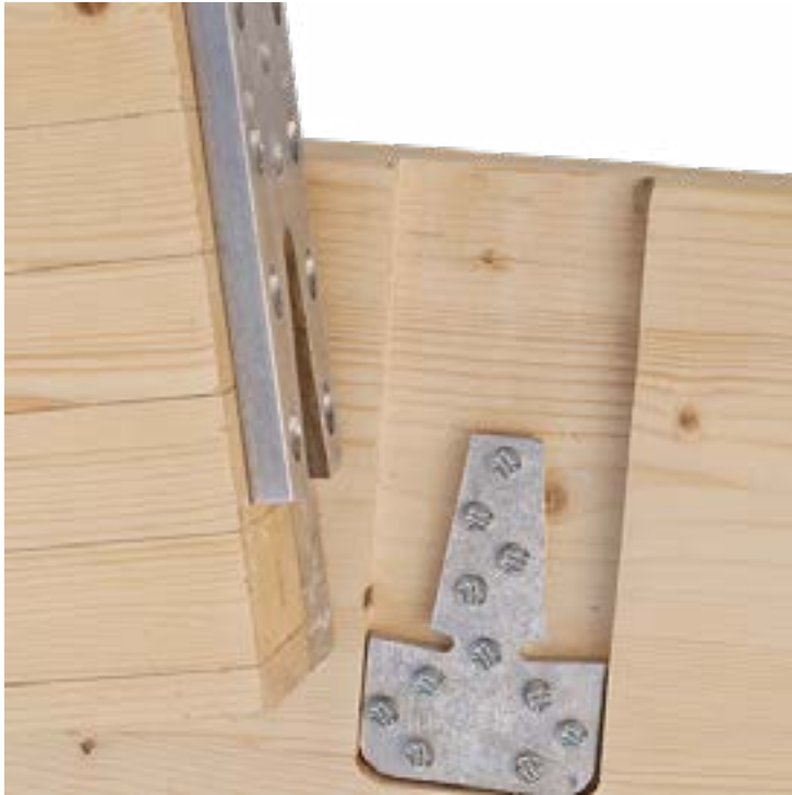
Invisible wood construction
