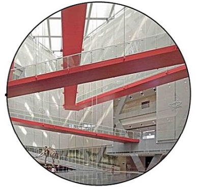
CONNECTING TWO SIDES OF THE BUILDING
