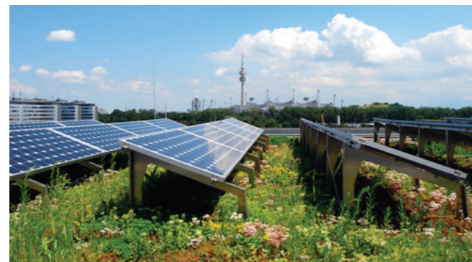
Fig. 15: Solar panels placed on an extensive green roof.
