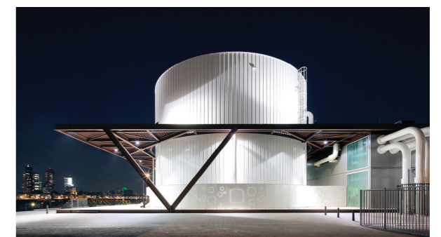
Fig. 20: Harbor-heat transmission station 'Warmtehub Brielselaan'.
