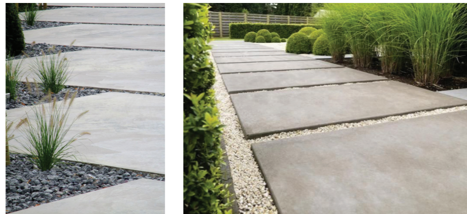
Fig. 12: Examples of one-on-one reuse of cut out silo walls as large pavement panels.
