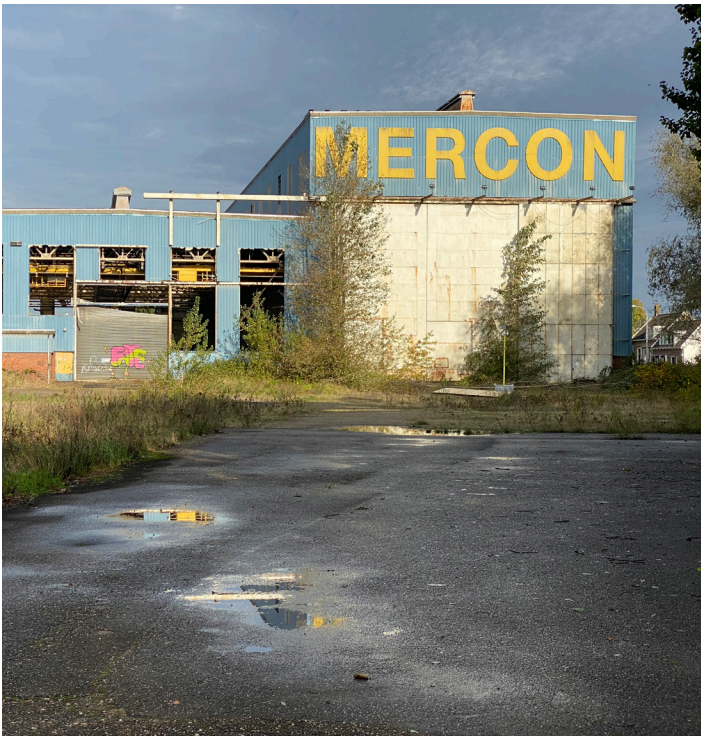
(Former) combination of brick & steel
