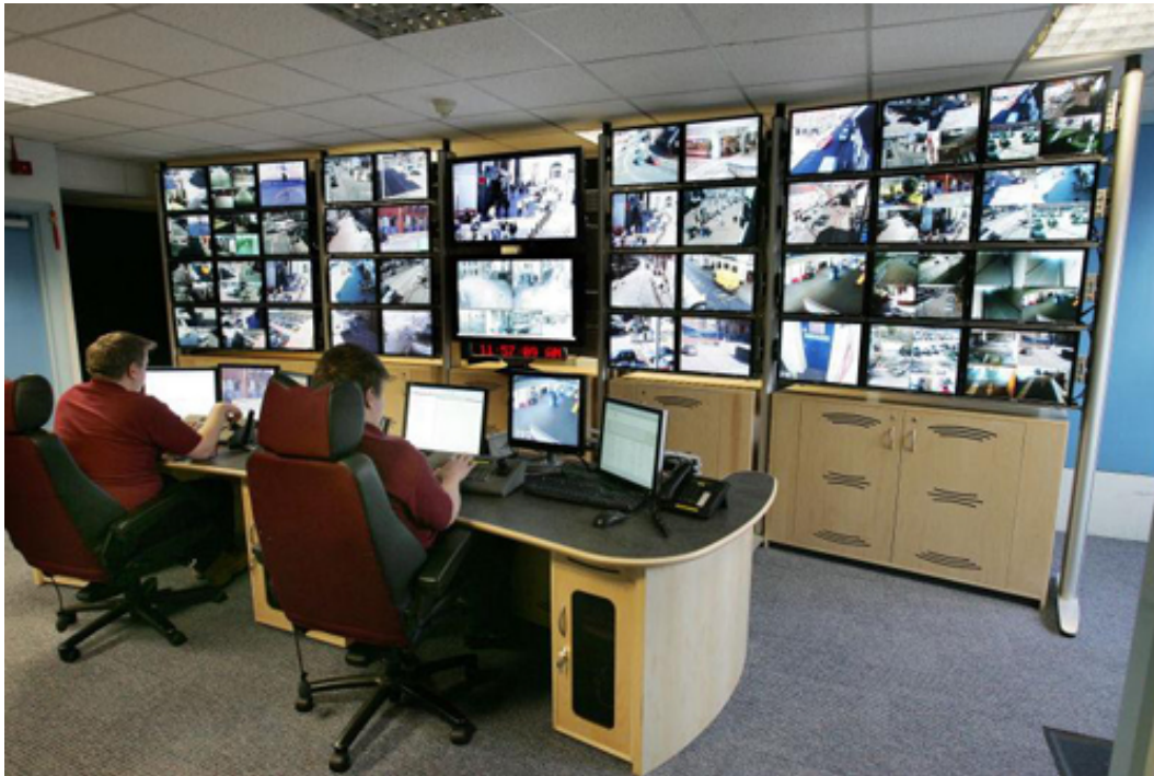
Figure 1.1: A matrix of CCTV monitors. Static monitors show the overview, a PTZ monitor stands in front of the operator. From http://ipcctv-solutions.com .
