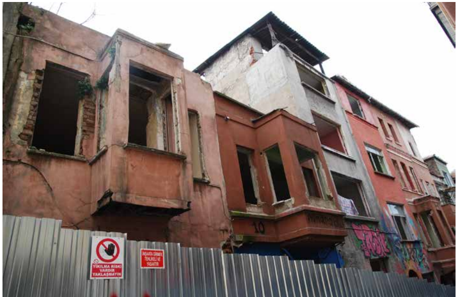
FIGURE 5.49 Empty buildings in Tarlabası after the evacuation, picture by the author.
