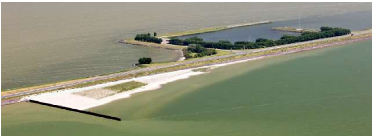
Figure 1-3 Overview Houtribdijk June 2016 with sections of vegetation. (source: recording of RWS Jurriaan Brobbel)
