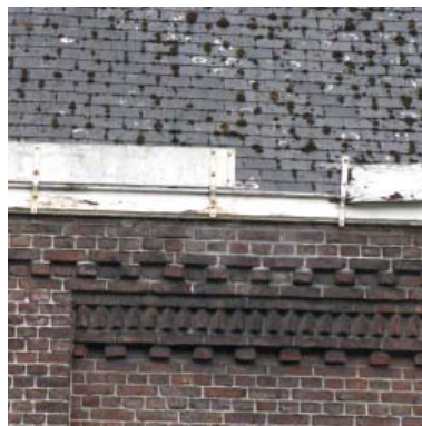
Figure 17. Bitumious slates and wood gutter
