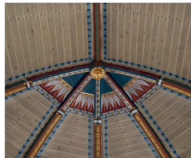
Figure 23. The paintwork of the vaulted ceiling; choir
