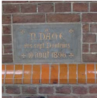
Figure 15. Glazed brickwork strip
