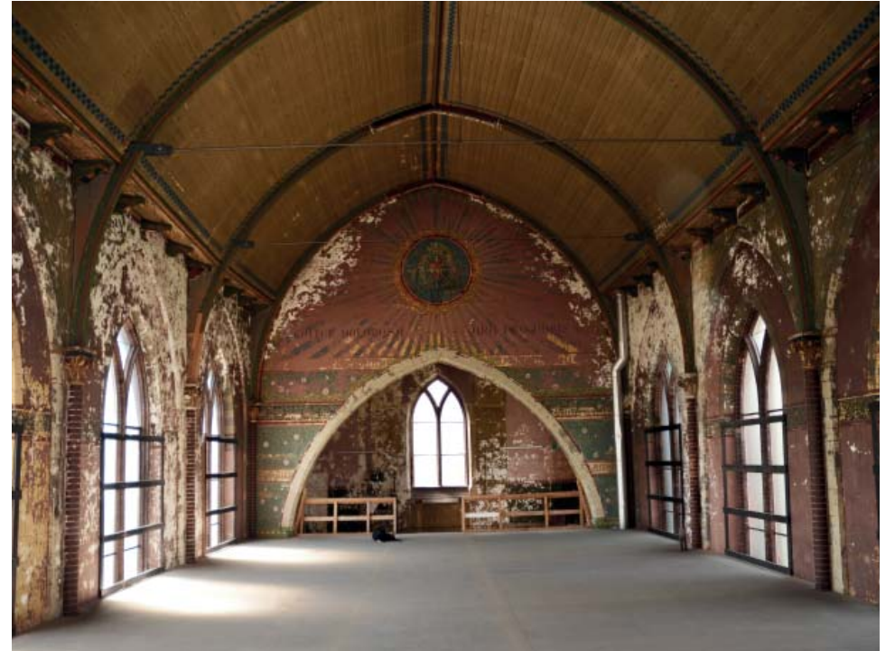
Figure 5. The first floor of the chapel; facing west
