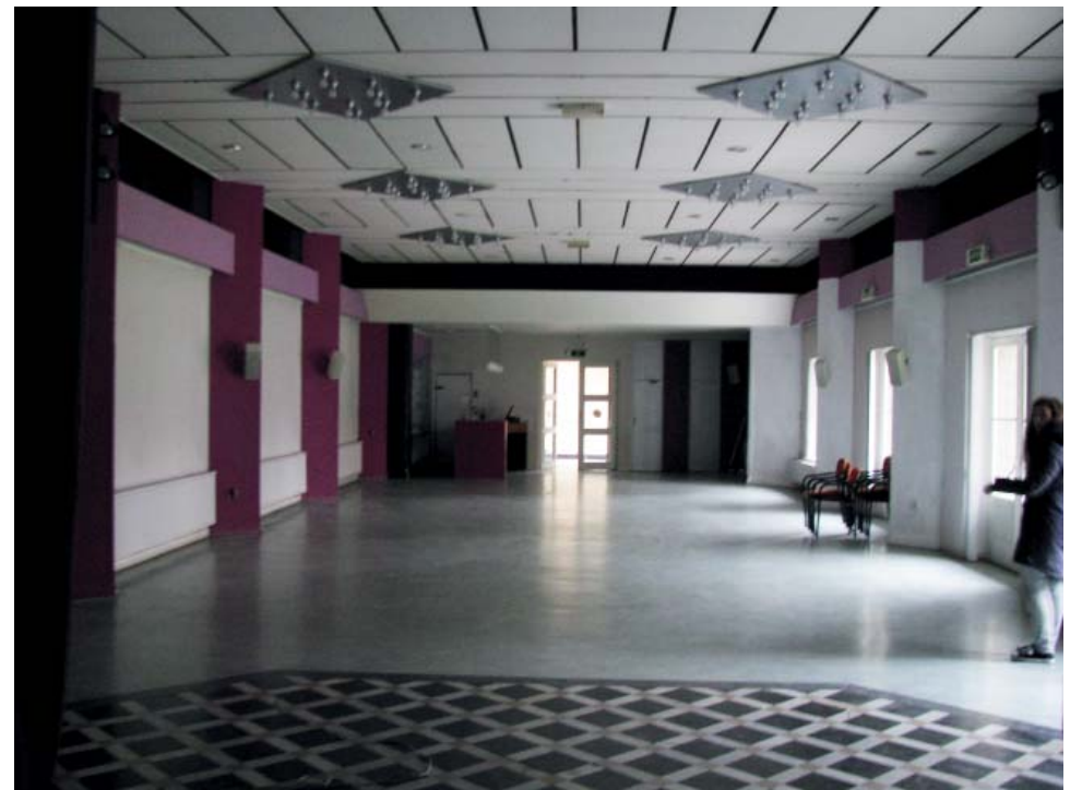
Figure 6. The ground floor of the chapel; facing west
