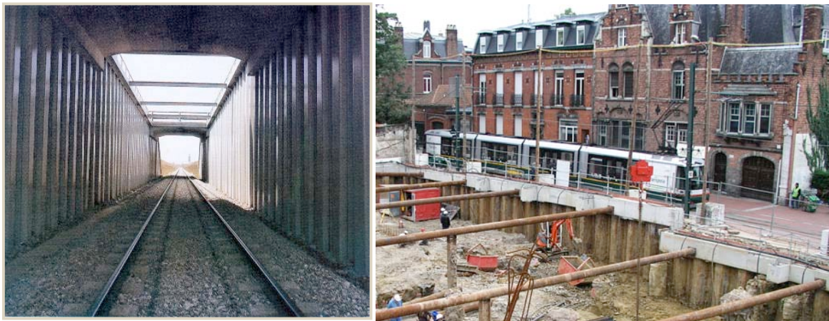
Figure 1. Sheet piling structures (underground car parks, tunnels, open-cuts, ...)
