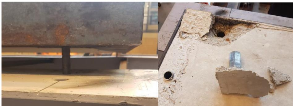
Figure 5.4: Damage due to placing deck (adapted from [21])
