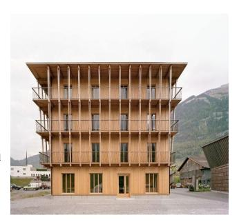
fireplace) with durability, while maintaining a minimalist aesthetic that resonates with Alpine vernacular architecture. The absence of insulation layers and reliance on solid timber walls challenge conventional energy efficiency norms, suggesting a climate-specific design strategy. Its emphasis on lifecycle thinking and adaptability provides a valuable case study for material-conscious, resilient architecture in Alpine contexts.
