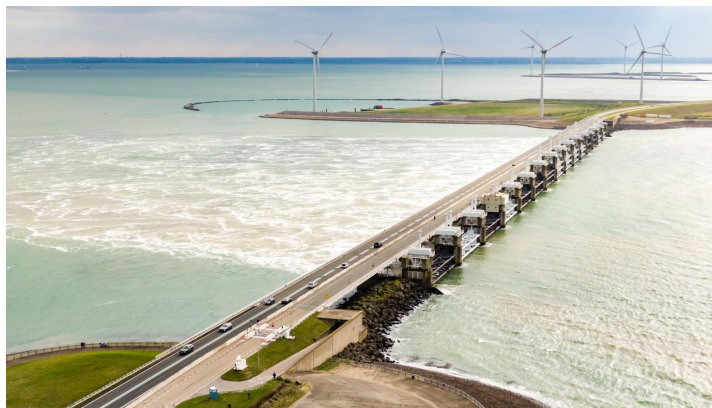
Figure 1.1: The Eastern-Scheldt Storm Surge Barrier. Source: https://www.nu.nl/binnenland/6029677/oosterscheldekering-gesloten-vanwege-hoge-waterstand.html .
