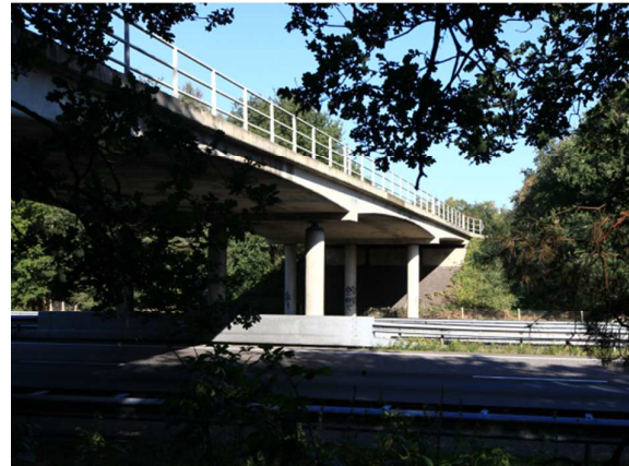
Figure 1. Viaduct de Beek
