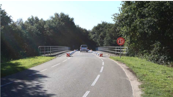
Figure 3. Traffic restriction on viaduct de Beek
