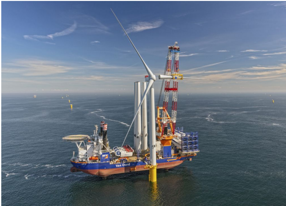
Fig. 4.15 – Coupling of the turbine blades with the nacelle from the Aeolus (HLV) self-elevating unit at Borssele III&IV offshore wind farm.
