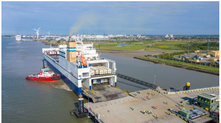
Figure 6: A view of unloading a Ro-Ro Vessel (Mandra, 2020)
