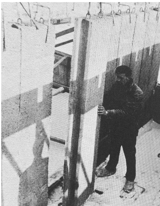
Figure 28: Simplex system. Reprinted from (Van Elk & Priemus, 1971)
