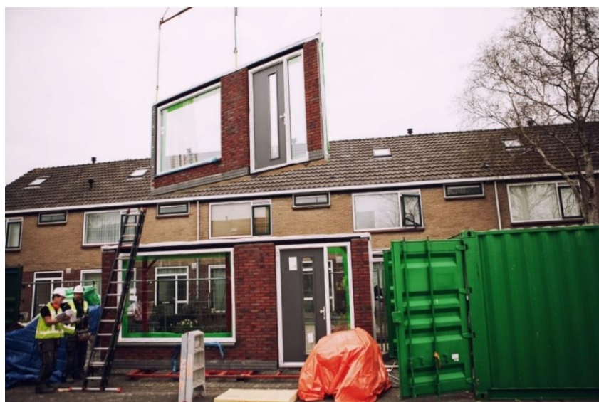
Figure 4: Prefabricated element on the building site (Akkerman, n.d.)
