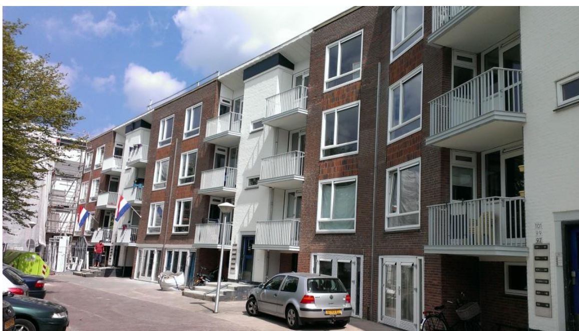
Figure 6: Renovated walk-up apartments in Zwolle (Stichting WE Adviseurs, n.d.)
