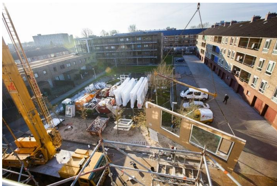
Figure 5: Prefabricated element (Dura Vermeer, 2015)
