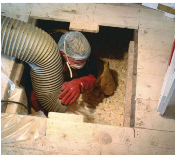
Figure 40: Chips for insulating the crawl space. Reprinted from (Traas Ongedierte Bestrijding, 2019)
