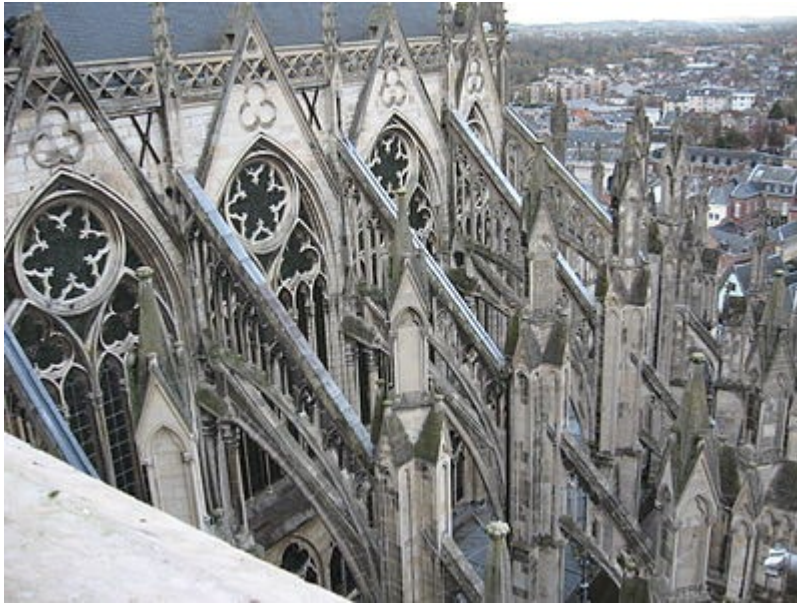
Figure 10: Flying buttresses, Amiens Cathedral, (Wikipedia contributors, 2025)
