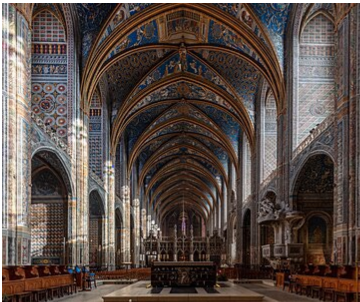
Figure 12: Rib vaulting, Albi Cathedral, (Wikipedia contributors, 2025a)
