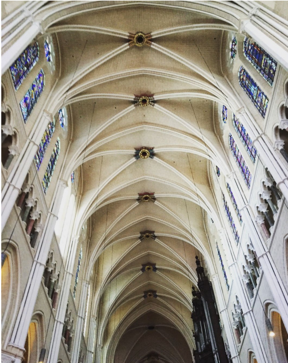
Figure 8: Rib vaulting Chartres Cathedral, (Jessiechensaid, z.d.)
