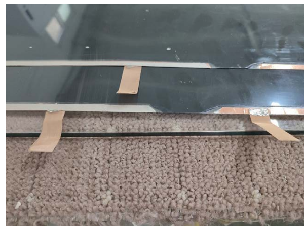
Figure 5: Preparing films for busbar installation.
