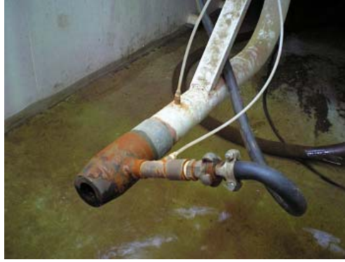
Figure 33 Detail of the water jet construction
