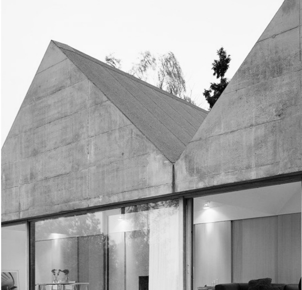
Roof reference: Summerhouse Lagnö
