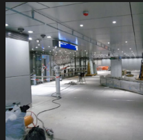
③ Access to Platform
