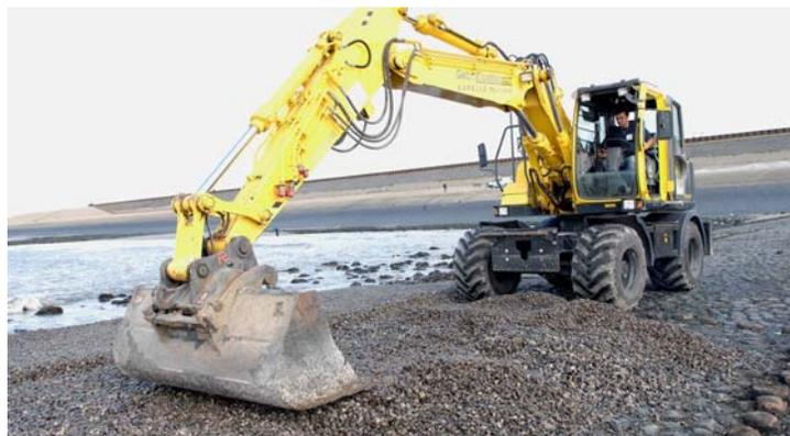
Figure 6.5 Profiling of freshly put Elastocoast with a hydraulic crane (photo: BASF Nederland B.V.).
