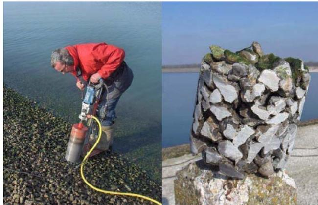
Figure 6.4 Drilling of core samples from an Elastocoast revetment (Bijlsma, 2008).
