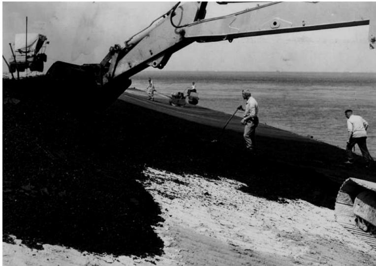
Figure 2.3 Application of an asphalt revetment on a dike (Verhagen, 2008).
