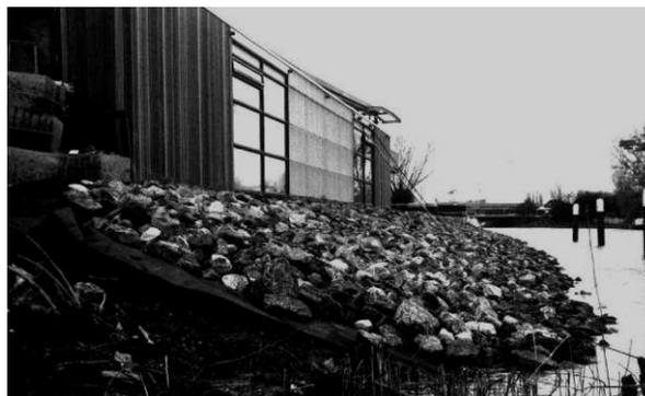
Figure 2.6 Dumped rock revetment (Verhagen, 2008).
