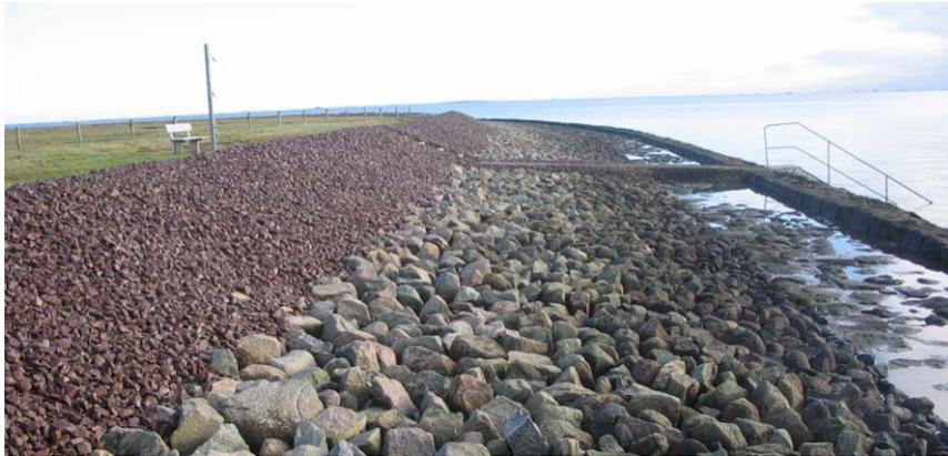
*Figure 1.2 German Elastocoast pilot on the island of Hallig Gröde. An Elastocoast cover layer has been placed on a breakwater on top of the revetment.*
