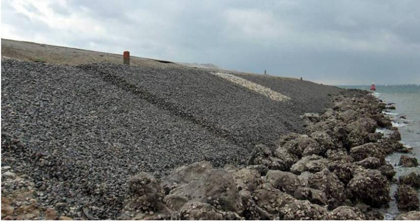
Figure 1.4 Dutch Elastocoast pilot at Ouwerkerk. The Elastocoast structure is placed on the slope of a rudimentary sea-dike in the Eastern-Scheldt.
