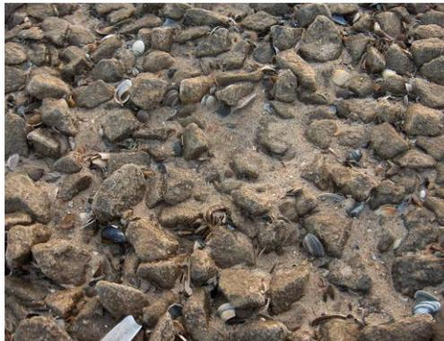
Figure 3.7 The Elastocoast pilot location Petten suffered from large amounts of sand and other abrasive material, but no extra damage was observed (Bijlsma, 2008).
