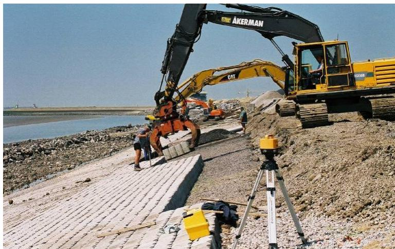
Figure 2.4 Mechanical placement of concrete blocks on a dike slope (Dorst, 2007).
