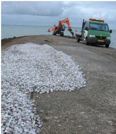
*Figure 3.1 Granular aggregate ready to be used for the Dutch Elastocoast pilot at Ouwerkerk.*
