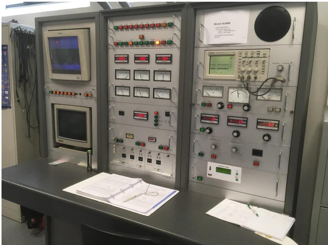
Figure 6.4: Monitoring and setup system for the van de Graaff electron accelerator
