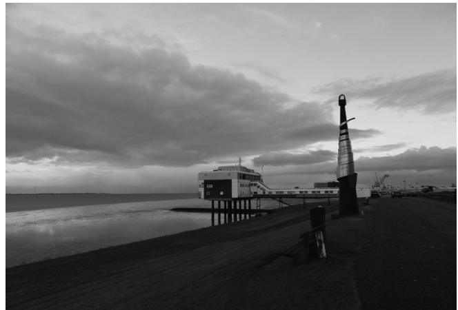
Illustration 1: The Dike of Delfzijl near the Eemshotel Source: Author
