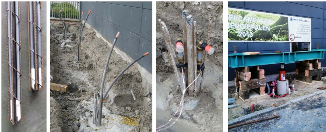
Figure 18: Energy piles installed for a BBRI test program in Ostend (Belgium). The heat exchangers are attached to the reinforcement cage prior to installation. The energy piles are fully monitored with strain and temperature sensors.
