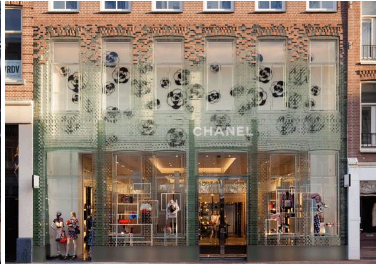
Cast glass façade for the Chanel Crystal house in Amsterdam. Retrieved from ABT (2016).
