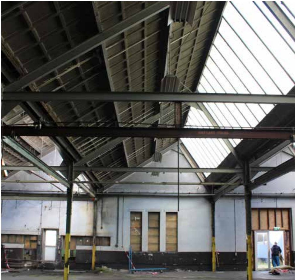
Fig. 5.3.1 Structure A (photo by authors)
