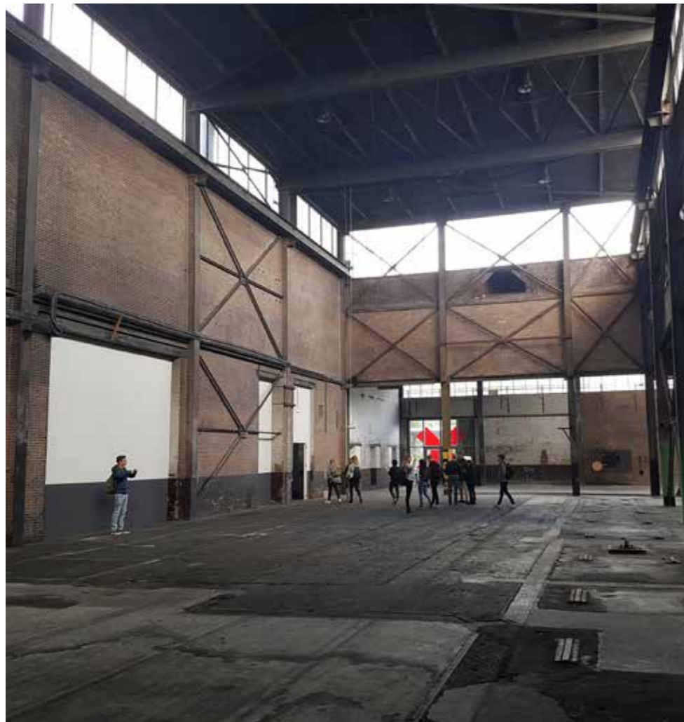
Fig. 5.3.5 Structure C1 (photo by authors)
