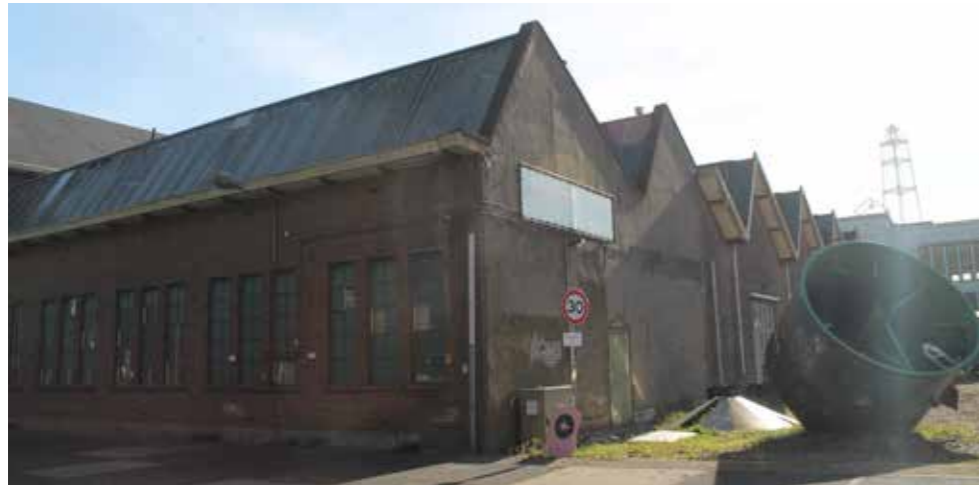
Fig. 3.4.1 Exterior building 333, characteristic saw-tooth roof
