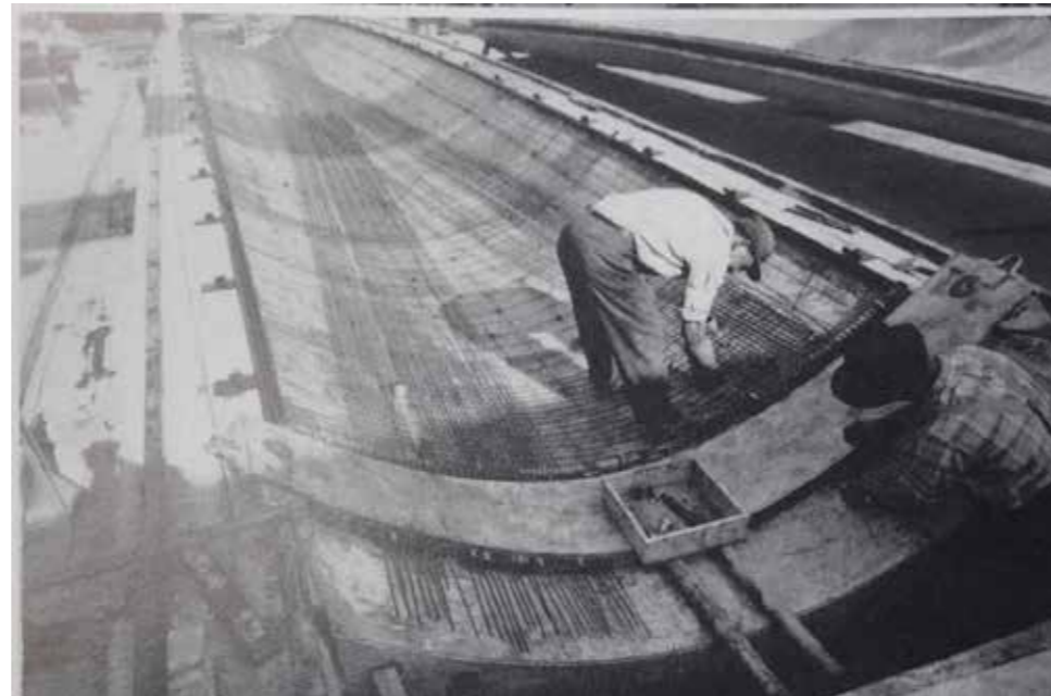
Fig. 5.5.9 adjusting the reinforcement Manual of Precast Concrete Constructions Vol. 1, p. 42
