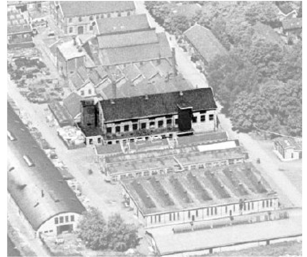
Fig. 4.9.3 original window openings east side 1932-1940 Photo: from collection Hembrug Museum
