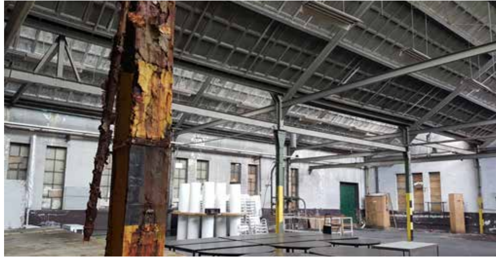
Fig. 3.4.2 Interior building 333, Bims concrete elements prominently present
