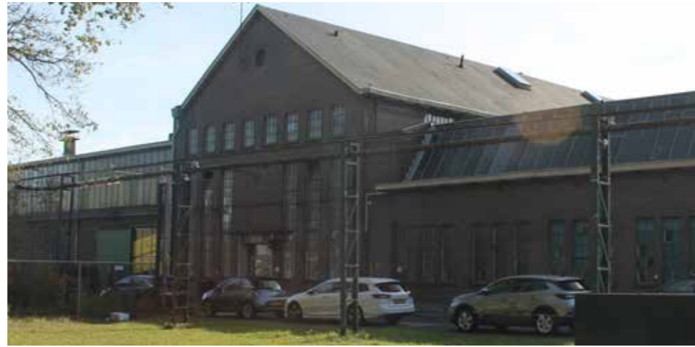
Fig. 3.4.4 Exterior building 72, gable roof drawing attention
