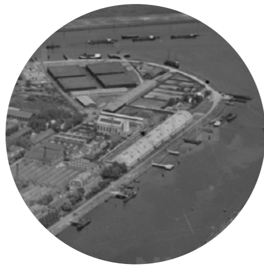
Demolishing of long Marine shed
