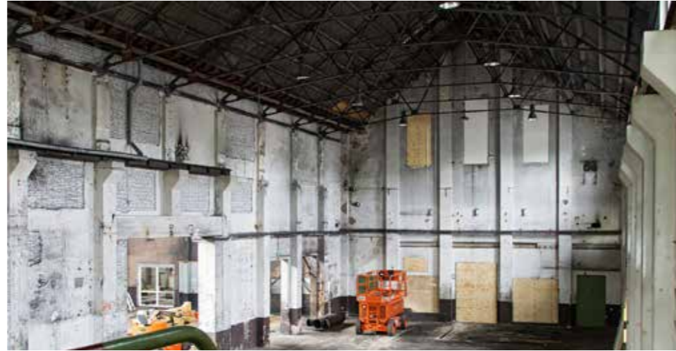
Fig. 3.4.5 Interior building 72, Visible gable roof structure and high ceiling
