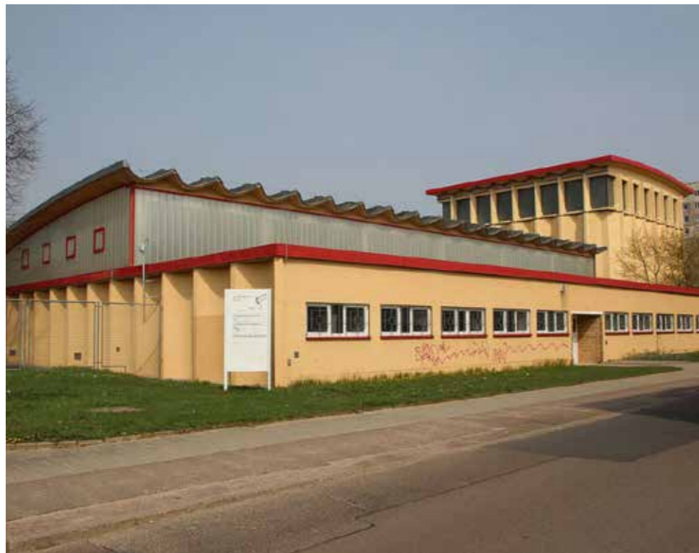
Fig. 5.5.17 Gymnasium, today the National Center for Rhythmic Gymnastics, Halle-Neustadt by Herbert Müller, Photo by Ralf Lotys, 2013.
