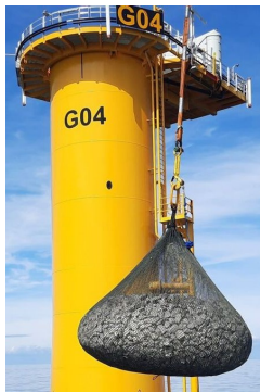
Figure 3.5: Suspended prototype scale rock bag
