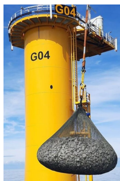
Figure 1.1: A rock bag is deployed near a monopile foundation (Ridgeway, 2024)
