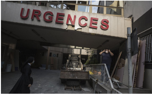
DAMAGED EMERGENCY SYSTEM
