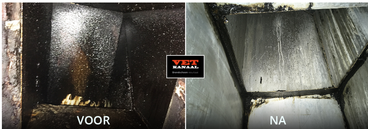
Figure 1-1: A comparison of an extraction channel before and after it is cleaned vetkanaal
