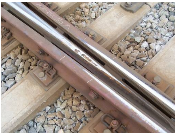
Figure 2 RCF damage of crossing nose
