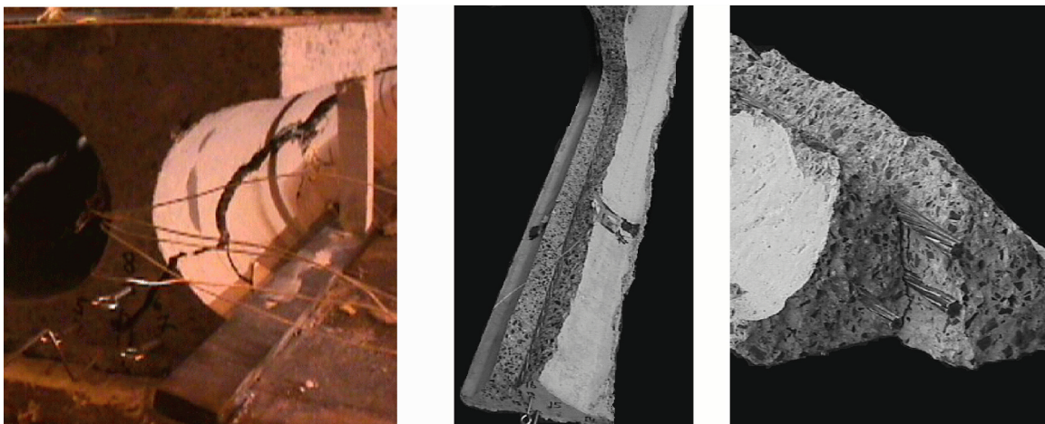
Figure 4.11: Details of the splitting cracks in VX265 specimen (left) and K400 specimen (middle and right) as observed after cooling down. In the middle figure one of the ribs is given from the support (lower side of the photo) to the loading point (upper side of the photo), right a detail of the cracks in the cover around the strands at the support.
