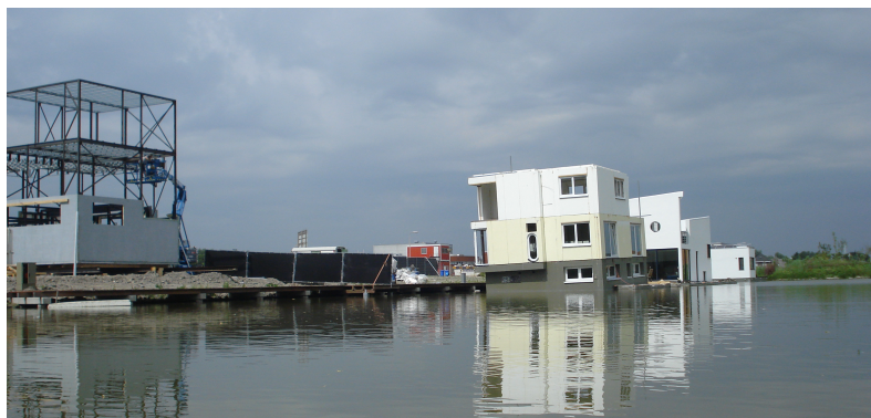
Figure 3.3: Floating houses in Harnaspolder.
