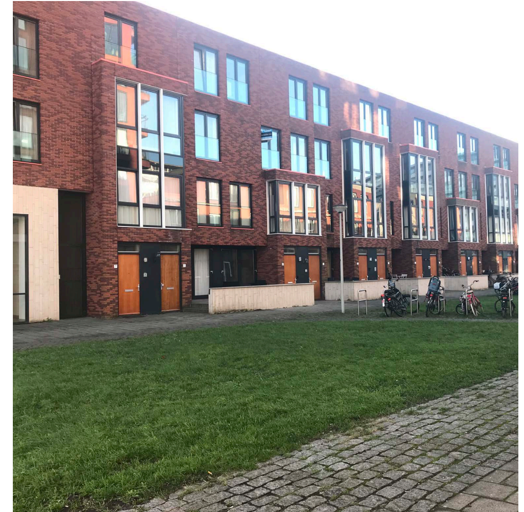
Houses connecting to groundflo No carparking in front of the living areas
