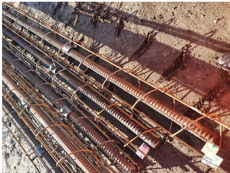
Figure 2.5: Example of how a tie-rod looks like in a rebar cage
