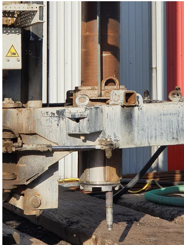
Figure 3.3: Pile grout delivery system for a SI pile
