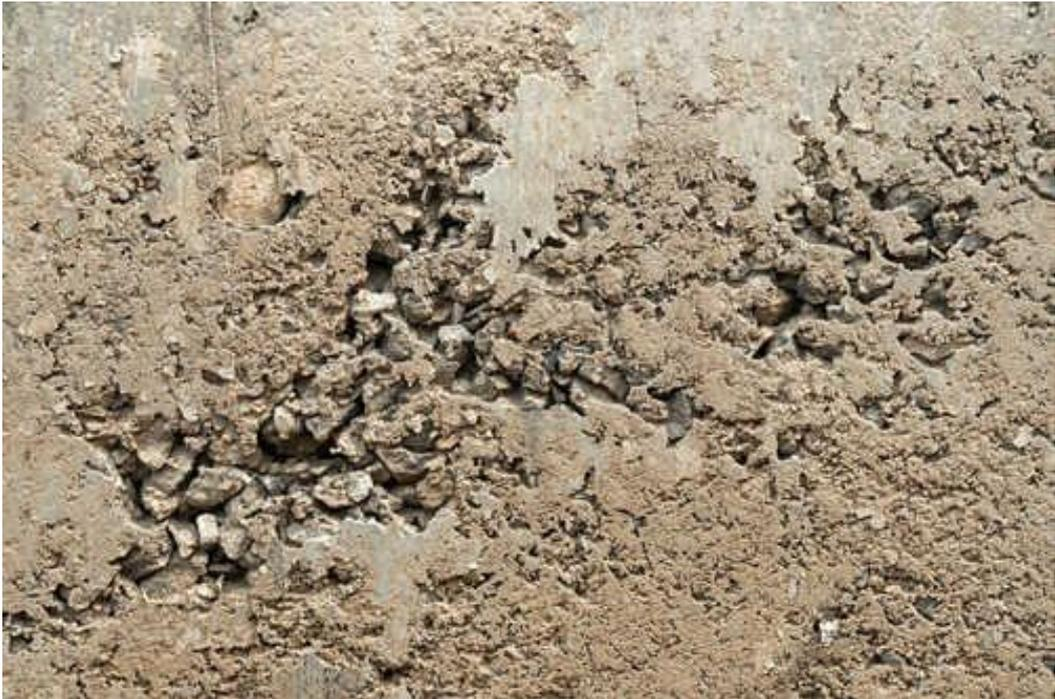
*Figure 5: Honeycombing visible on a concrete element [38]*
