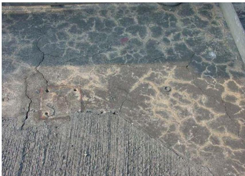
Figure 3: Concrete failure due to Alkali Aggregate Reaction [28]
