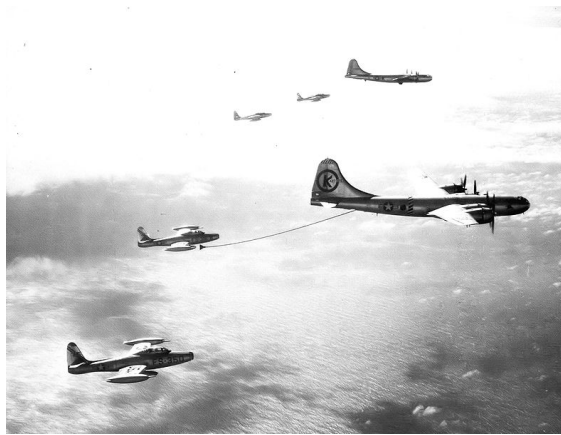
Figure 3.4: 43rd Air Refueling Squadron KB-29M Superfortresses refueling 48th Fighter Wing F-84s over the Philippines, 1953 [7]
