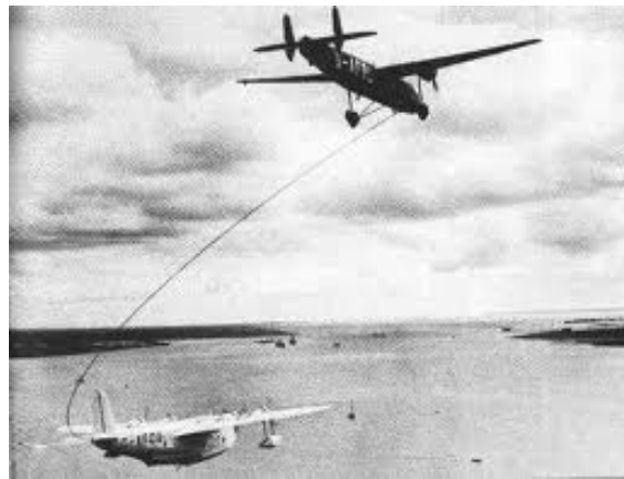
Figure 3.2: Flight Refuelling Ltd operated four Harrow tankers. One, shown here, 'tops up' an Imperial Airways 'C' Class flying-boat over Southampton's dock area prior to the non-stop transatlantic air mail service in 1939 [6]
