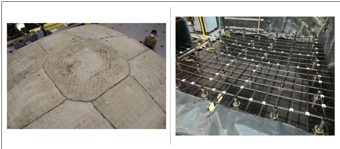
Figure 11. Prefabricated segments assembled into a whole shell (left); Reconfigurable mould actuated by a set of vertical mechanically driven pins and connecting flexible formwork (right). Photo credits: ©Robin Oval.
