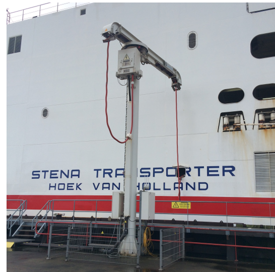
(b) The Cavotec crane in Hoek van Holland to provide shore power to the Stena Line vessels.
