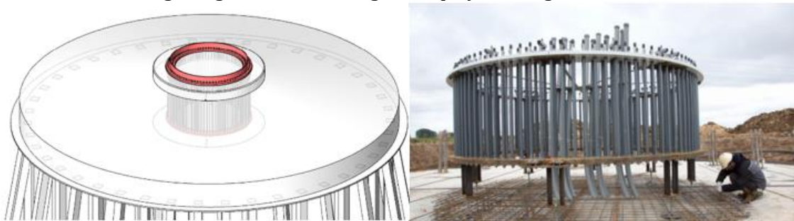
Figure 1-2a: Placement anchor cage; b: Impression anchor cage
