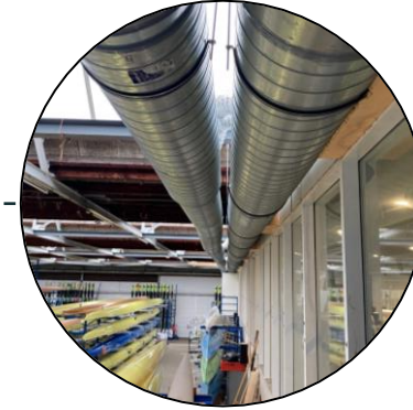
Balanced mechanical ventilation
