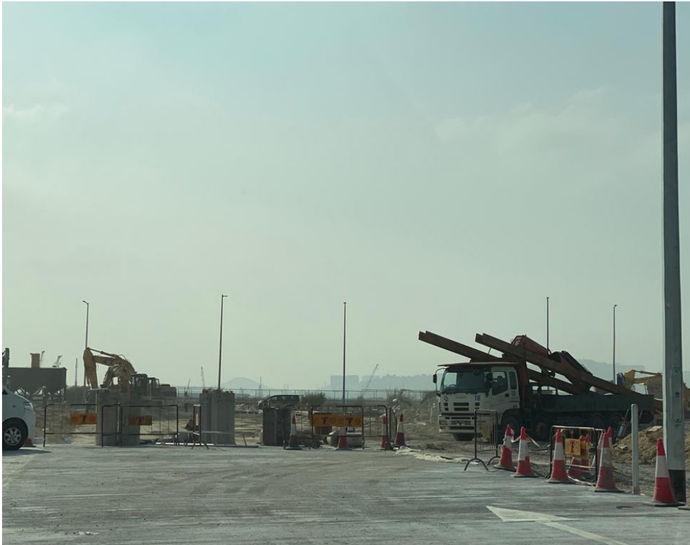
Figure 38. Construction site (road construction) on reclamation in Zone A. (Own photo, 2020)
