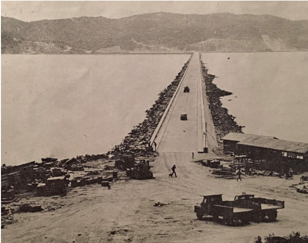
Figure 36. "Building of the isthmus connecting Taipa Island to Coloane Island". 1971, unknown author. https://www.reddit.com/r/OldPhotosInRealLife/comments/j4u8qf/macaubefore_and_after_the_cotai_strip/
