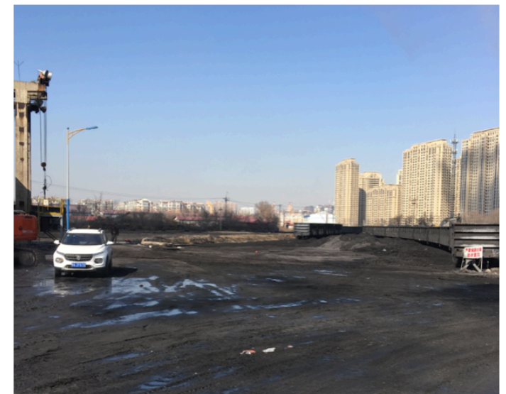
The coal-storage area
