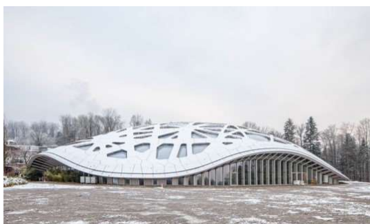
(a) Overview of the shell roof with the skylights
