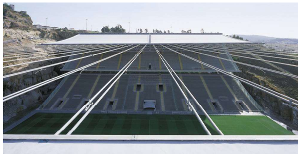
(a) Detail of the cables in the finalised roof structure
