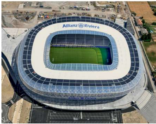
(a) Roof membrane existing of photovoltaic panels for generating electricity, PVC foil for shade, and ETFE foil for transparency
