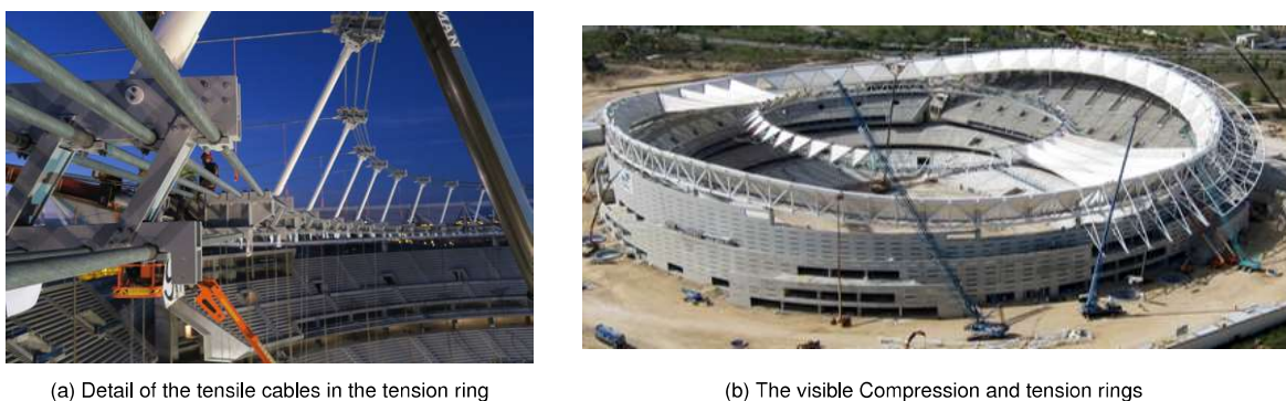
Figure 2.16: Structural system and the building process
