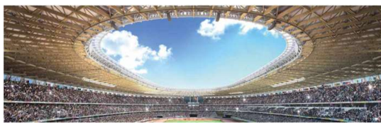
(a) View of the hybrid roof structure
