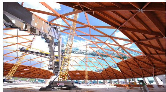
(b) Construction phase of one of the two geodesic dome structures
