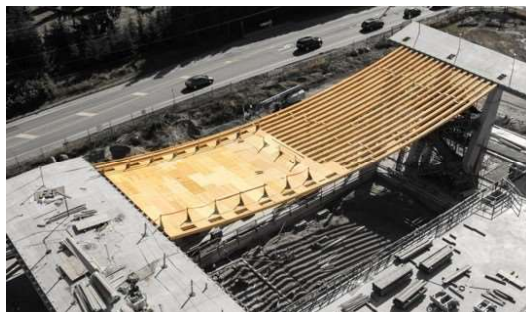
(a) The roof structure during construction
