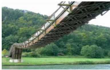
(a) Essing bridge in Essing
